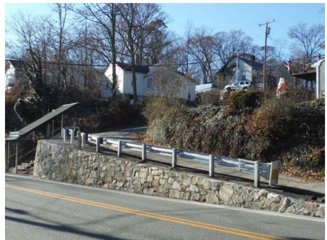
CR-609 Guide rail completed and road opened.
