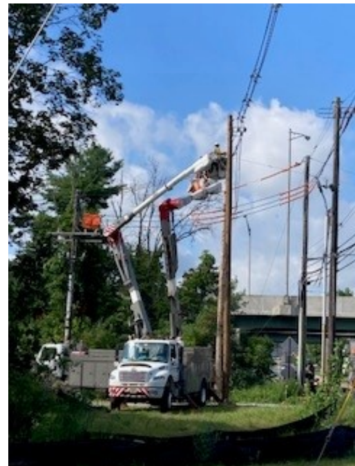
JCP&L Crew Installing Lines on New Poles
