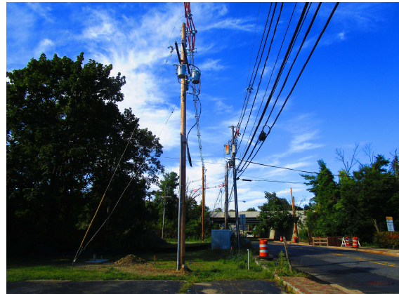
New Pole Line Installed to Accommodate Widened Bridge Structure
