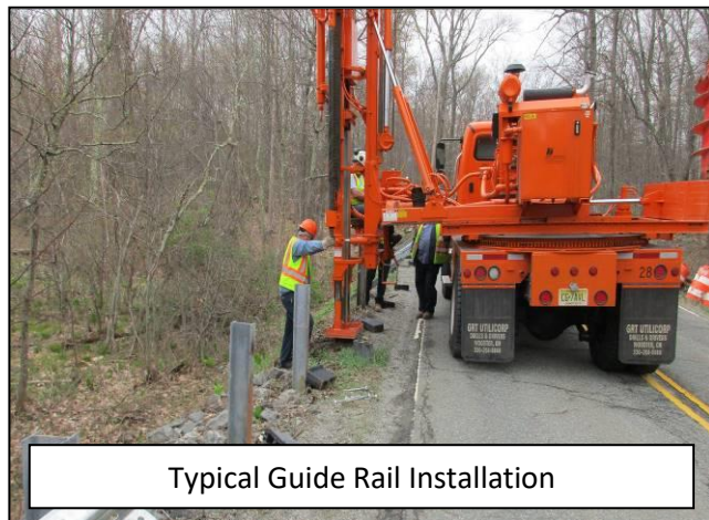
Typical Guide Rail Installation
