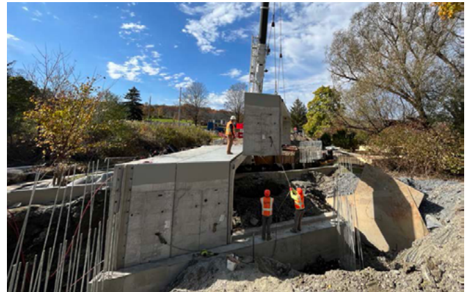
Installation of Precast Concrete Rigid Frame (Bridge) Segments
