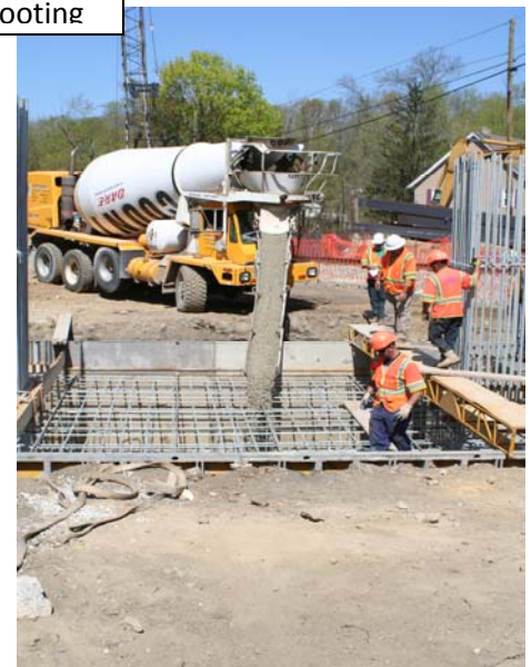
Pouring concrete at Pier 4 footing
