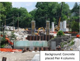
and Pier 3 South column Foreground: Concrete formwork in place for Pier 2 columns
