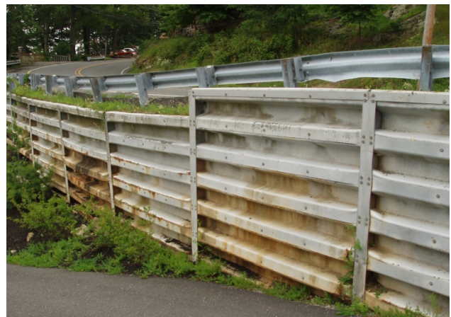
Picture of CR 607 Retaining Wall
