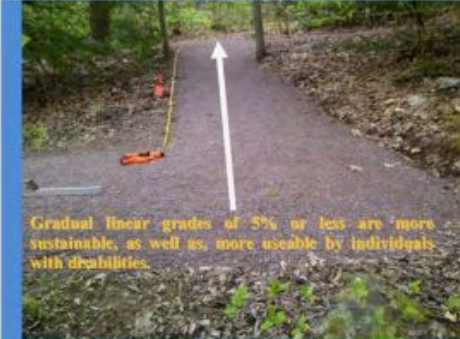
Figure 1: Measuring Linear Grade (Running Slope) of an accessible trail. © photo 2013 Penn Trails LLC
