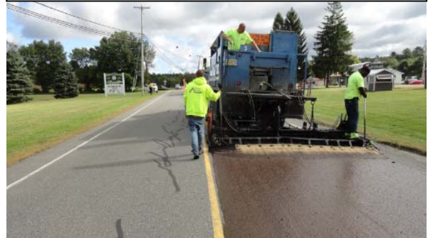
Typical Micro-surfacing Operation
