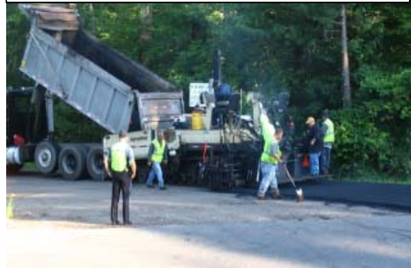
Typical Resurfacing Operation
