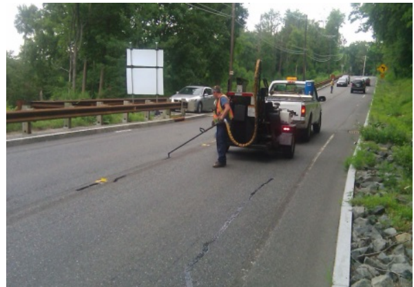
Typical Cracksealing Operation
