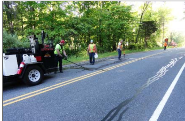
Typical Crack Sealing Operation
