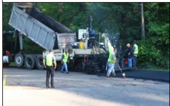
Typical Resurfacing Operation
