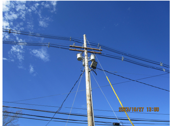
JCP&L Lines & Transformers Moved to New Pole
