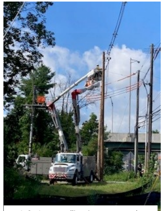
JCP&L Crew Installing Lines on New Poles
