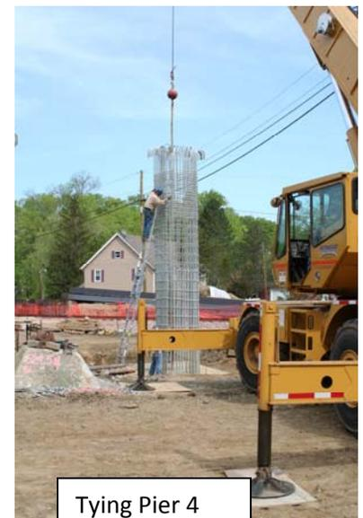
Tying Pier 4 column reinforcement
