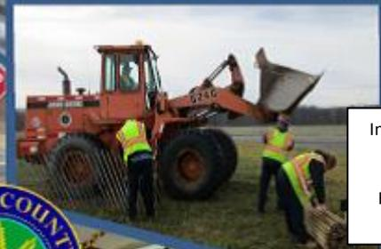
Installing snow fence in approved property lining the County’s Roadways to prevent snow drifts.
