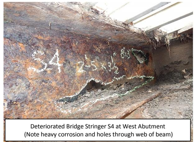
Deteriorated Bridge Stringer S4 at West Abutment
