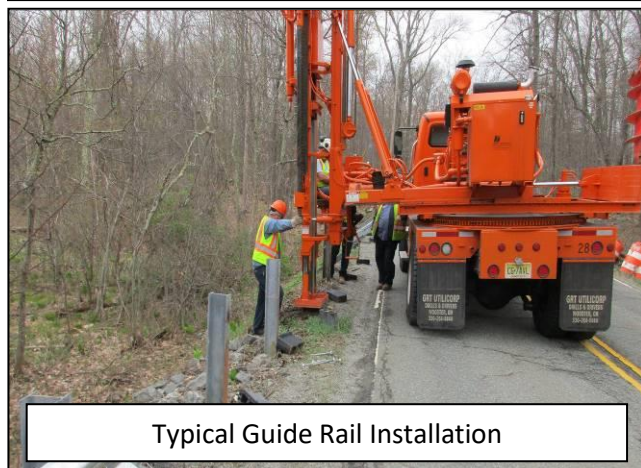
Typical Guide Rail Installation
