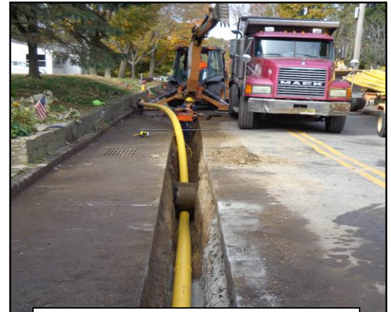
Roadway View: Typical Gas Main Pipe Installation
