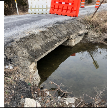
Upstream Fascia after Headwall Failure
