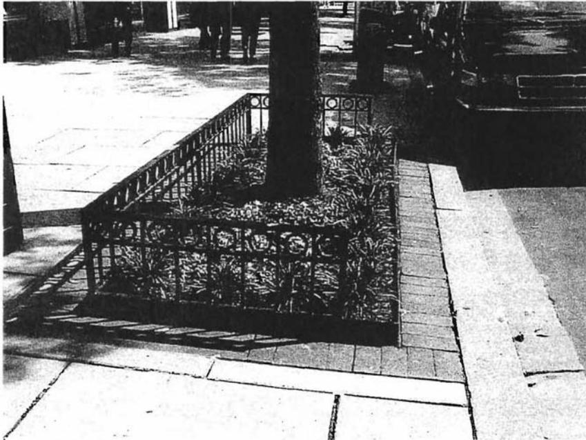
Figure 1. Tree pit with railing.
